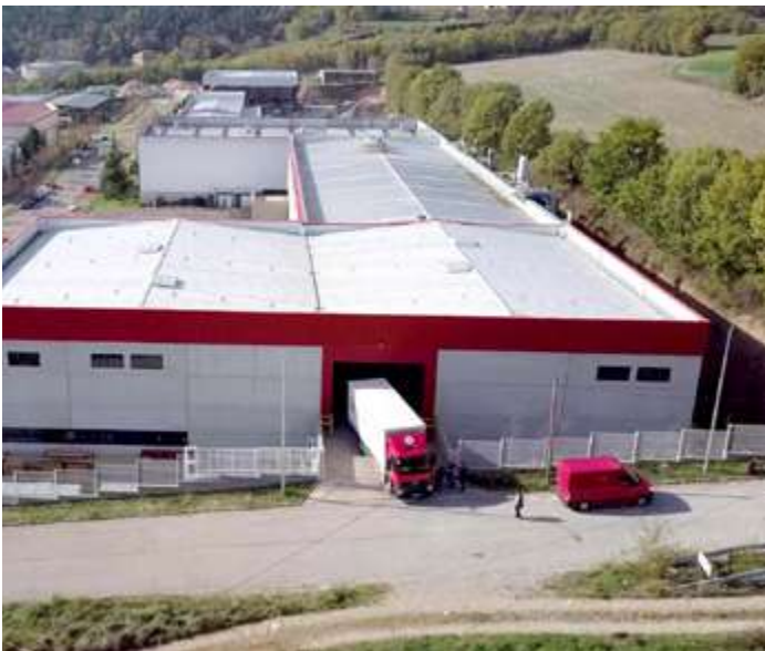
Technical textiles plant. Berga, Barcelona.
